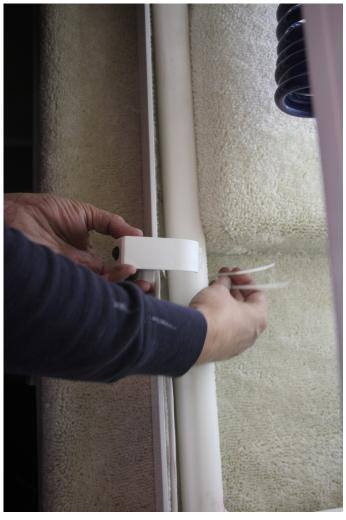
Clip the switch pod to the PVC downpipe just inside the door.
