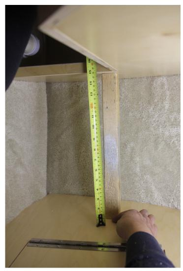
Use some sort of straight edge to determine where the long central support (with your light) will touch the closet floor. Go back about 1.25 inches and mark that point.
